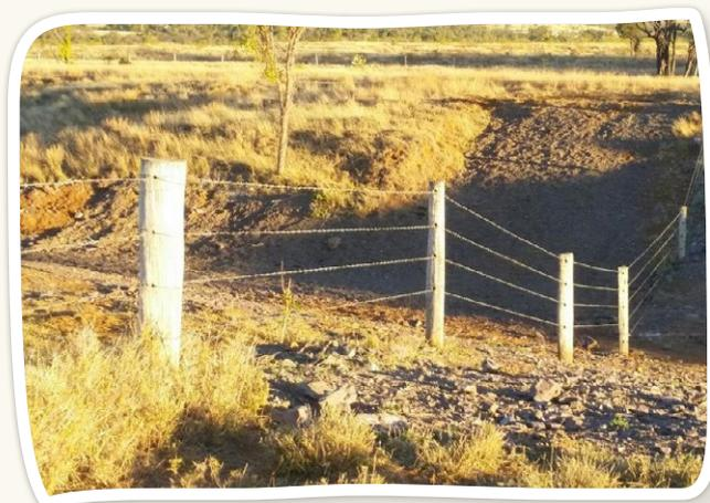
*A rock chute, constructed by landholders working together and with help from FBA, was so effective in addressing the problem that it withstood the impacts from Severe Tropical Cyclone Marcia in February 2015, with no erosion occurring at all.*
