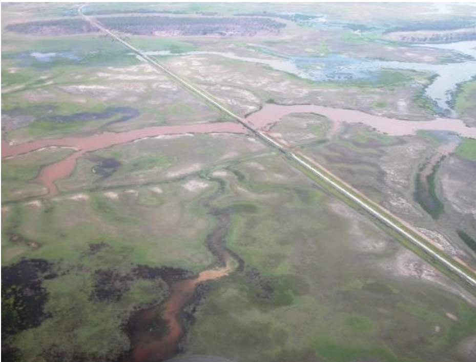
Figure 4.41. Railway embankment across wetlands at St Lawrence. Photo Roger Jaensch.
